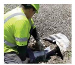
Designed to pry or cut the steel from mangled automobiles, we're probably the only government organization to use the Jaws-of-Life to straighten the crushed ends of steel culverts. Arapahoe County Road and Bridge partnered with Byers Fire Department and together they were able to turn an ingenious idea into a time- and cost-saving reality.
